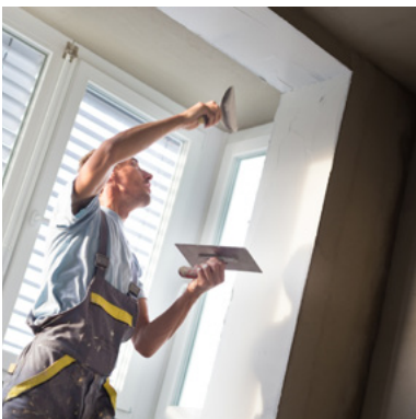
Protection during plastering
